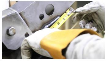
Within that zone, mark off how much frame you wish to remove, while still retaining a safe amount to weld with.
