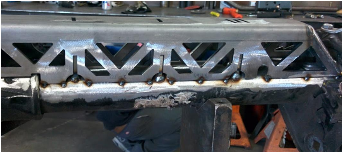
Figure 13. Back side of Truss Tacked
