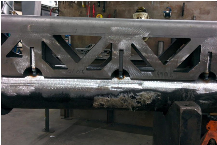
Figure 9. Center Plates Tack Welded
